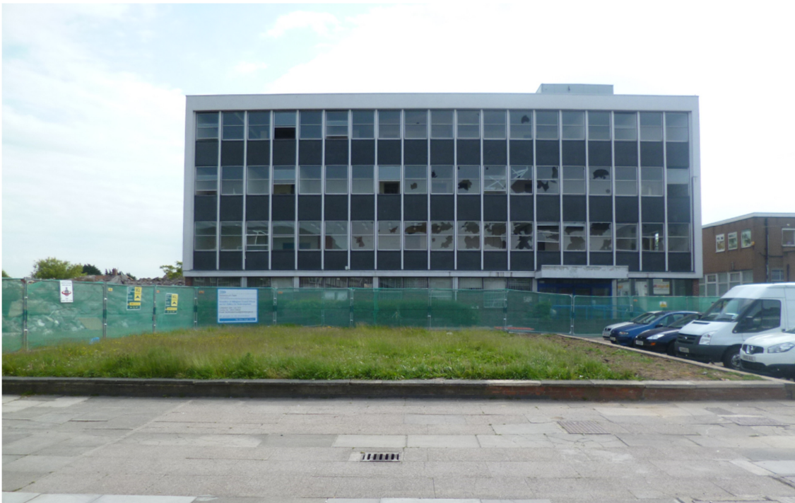
View from north to south to remaining council offices building
