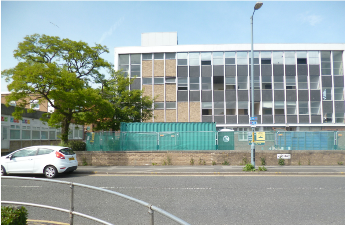
View from south (Grampian Road) to north
